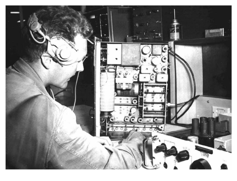
This picture shows radio technician servicing a Collins 51-J4 receiver in one of two screened rooms in the radio workshops section of the main operations building.
